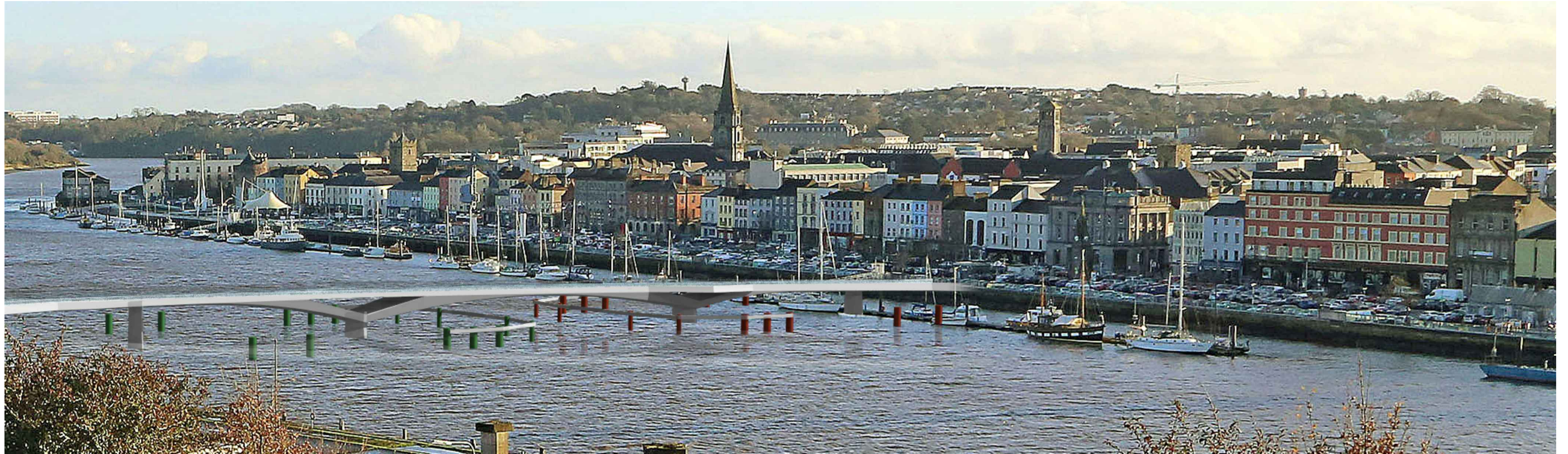
VIEW OF BRIDGE AND VESSEL COLLISION PROTECTION FROM NEAR ARD RI
